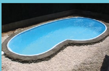
Assise beton - margelles
